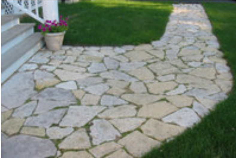
Figure 47 A broken flagstone pathway Retrieved from: myhomeredux.com
