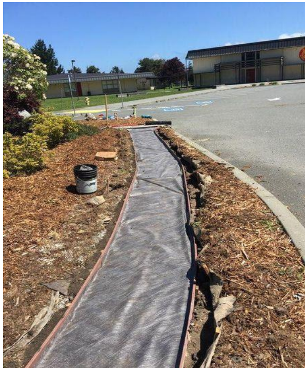
Figure 3: Area prep for permeable concrete, Zane Middle School (Sicaud 2018)
