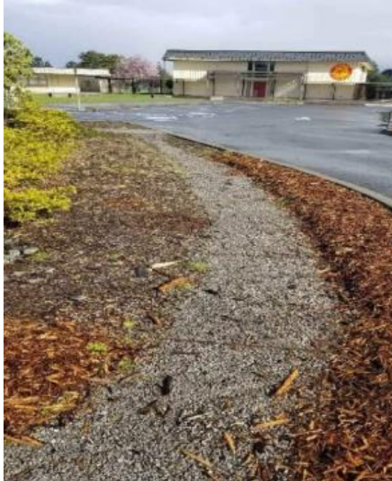
Figure 22 Path that needed to be redone
