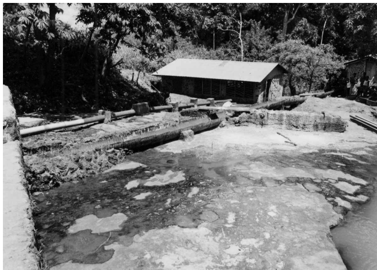
Figure 3. Cofferdam, head gate and penstock leading into turbine house. Photograph by author, near Boyangana, 1995
