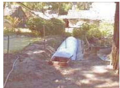
Photo 92. Make a system so the rain water is led away.
