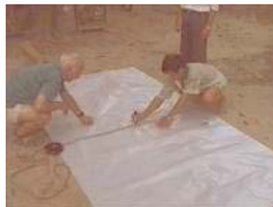
Photo 13. Marking the place to cut the plastic
