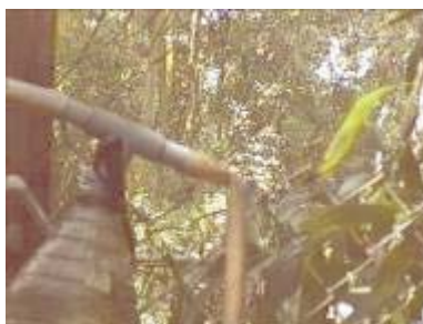
Photo 76. Hose pipe bent down (#4) Cut the damaged hose and join it again
