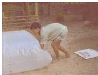
Photo 36. Forcing the air from the 3m tube to the main tube
