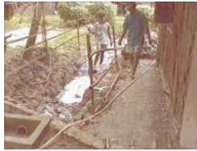
Photo 88. Starting to fix the trench
