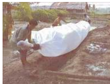
Photo 40. Placing the digester in the trench
