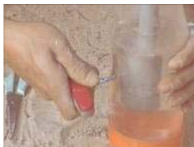
Photo 47. The PVC pipe is inserted into the bottle and a little hole is made to fix the water level
