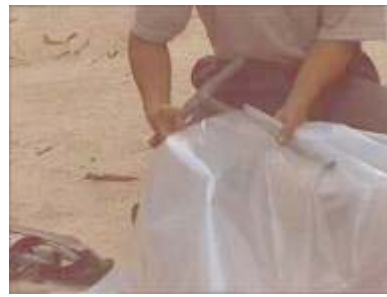
Photo 54. Placing the PVC "T" at the other end of the 3m plastic tube (one of the end of the "T" is joined to the hose coming from the digester and the other to the stove)
