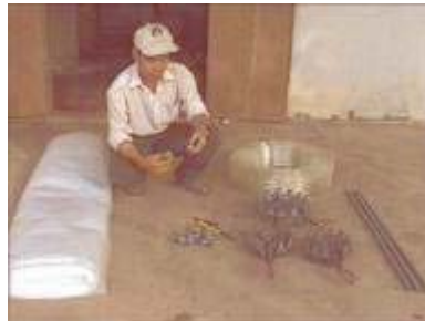
Photo 11. Materials for installing a plastic biodigester
