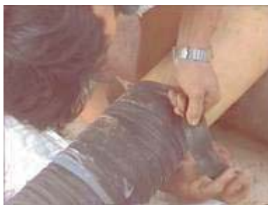
Photo 24. Completing the wrapping of the plastic over the inlet pipe
