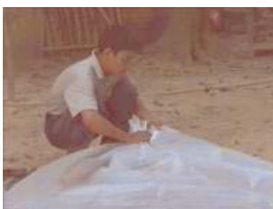
Photo 51. Closing one end of the 3m plastic tube
