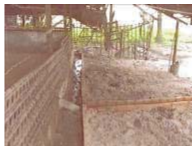
Photo 71. After placing the digester
