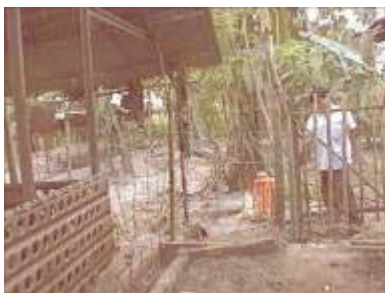
Photo 68. Fencing around the area where the biogas digester is located
