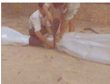
Photo 33. Tying the 3 m length of plastic tube to the exit pipe
