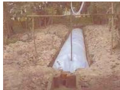
Photo 67. The finished installation
