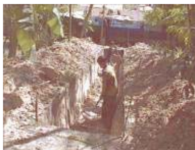
Photo 5. Excavating the soil
