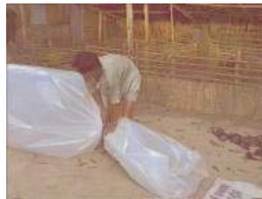
Photo 30. Tying the tube but leaving enough plastic to insert the outlet pipe
