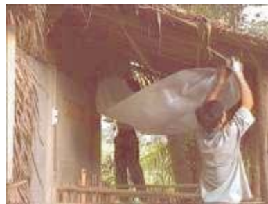
Photo 58. Suspending the reservoir bag in the roof space
