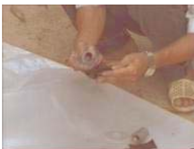
Photo 16. Preparing the materials for the gas outlet
