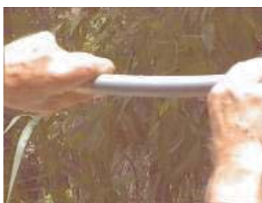
Photo 79. Make a hole in the PVC pipe, take the water out and stick it again with tape or a rubber band (# 6-2)
