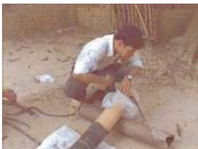
Photo 25. Covering the entrance of the inlet pipe with a plastic bag
