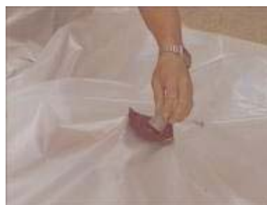
Photo 17. Tightening the gas outlet (without using glue)
