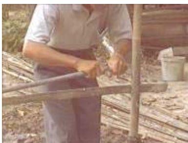
Photo 43. Connecting a plastic hose (or rigid PVC tube) to the PVC gas outlet
