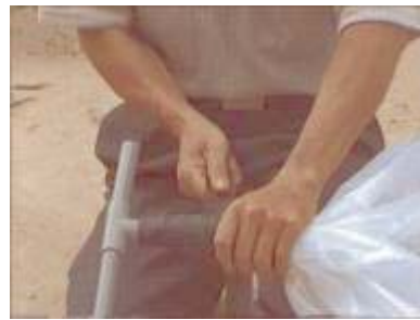
Photo 54. Placing the PVC "T" at the other end of the 3m plastic tube (one of the end of the "T" is joined to the hose coming from the digester and the other to the stove)
