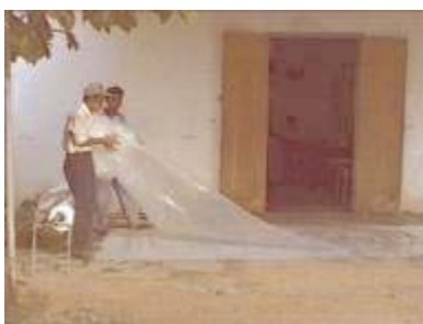
Photo 8. Bundling one plastic tube in preparation for putting it inside the other
