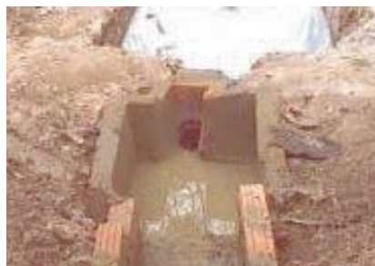
Photo 91. Make a system to capture the sand in the inlet box
