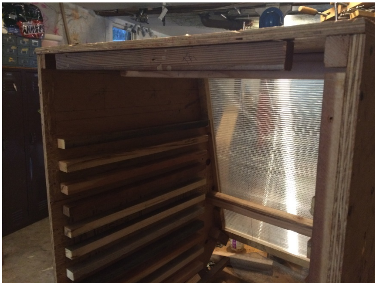
Figure 5-7 Weather proofing and Door fitting
