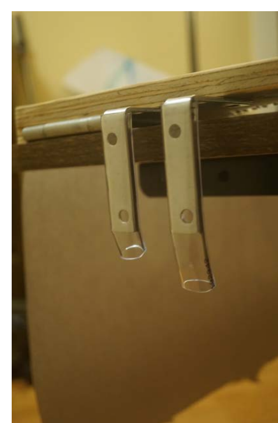
A: Metal L-Brackets preventing over-extension and enhancing durability.
