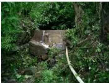
Hydro installation in Honduras (V. Grau)
