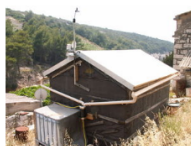
Dew collection roof retrofit
