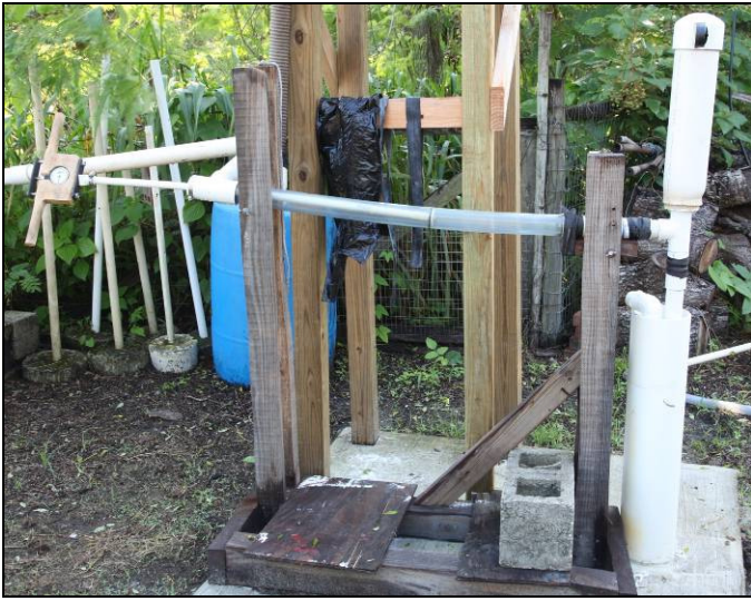
Rower pump with 27' suction pipe in borehole
