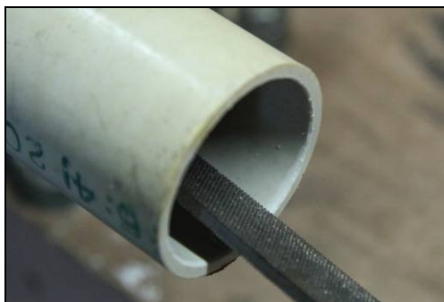
Filing the inside edge of a pipe
