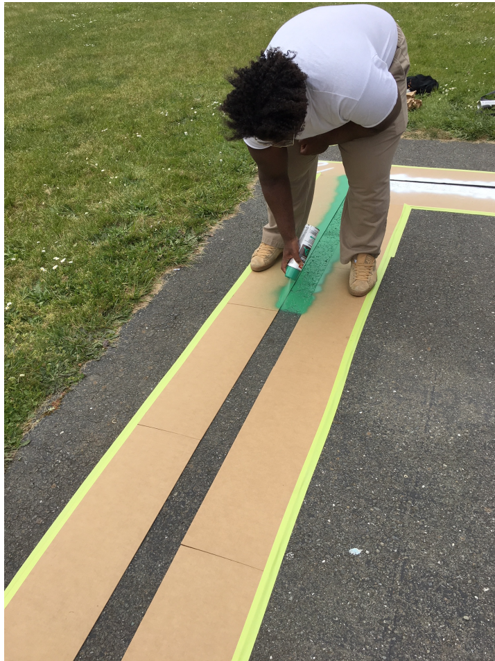
Figure 5-5: Using cardboard and tape to create a straight line (R. Turlington, unpublished photos, April 2018)
