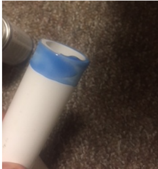
Figure 5-8: PVC glue applied to the end of a piece of PVC pipe (I. Duque, unpublished photos, April 2018)
