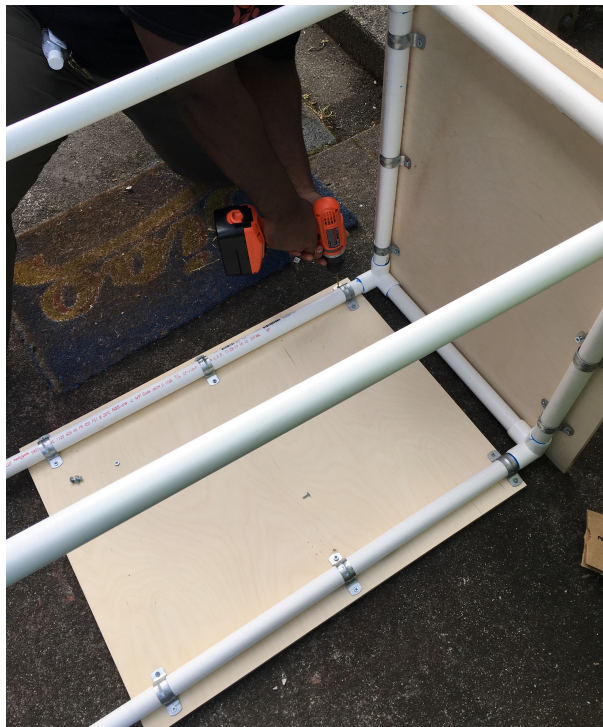
Figure 5-9: Securing the wood panels to the outside of the PVC frame (R. Turlington, unpublished photos, April 2018)
