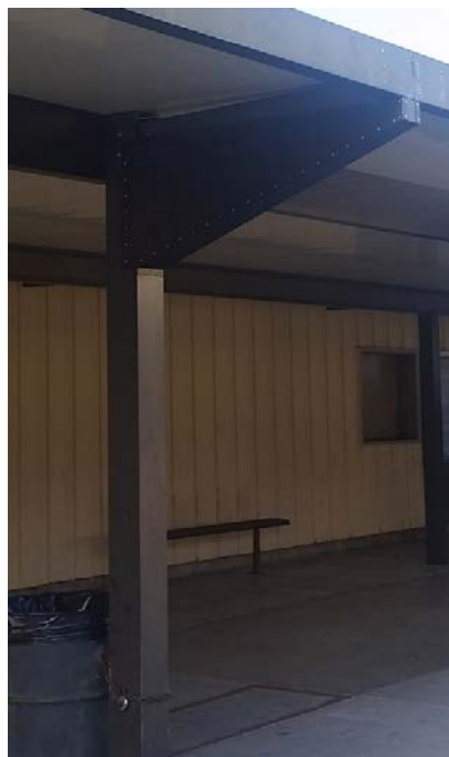
Figure 12: Streamline integrated gutter box installed at Zane Middle School.
