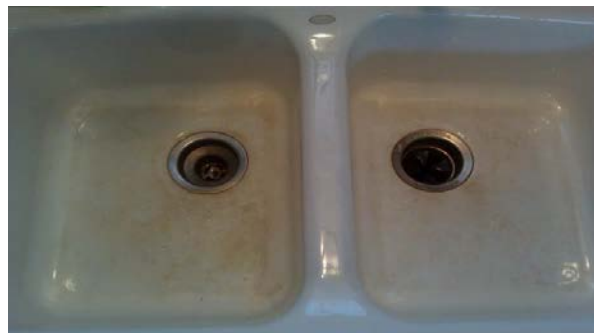
Figure 2.10.2: Reveals hard to remove stains on a basic porcelain sink.
