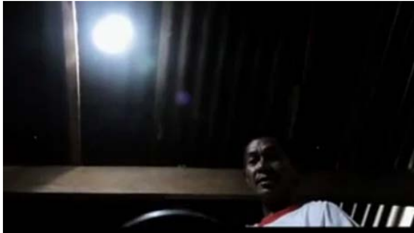
Figure 2.9.2: A skylight made of a plastic bottle is used inside a Philippine home. ( http://phys.org/news/2011-09-bottle-brighten-millions-poor-homes.html )
