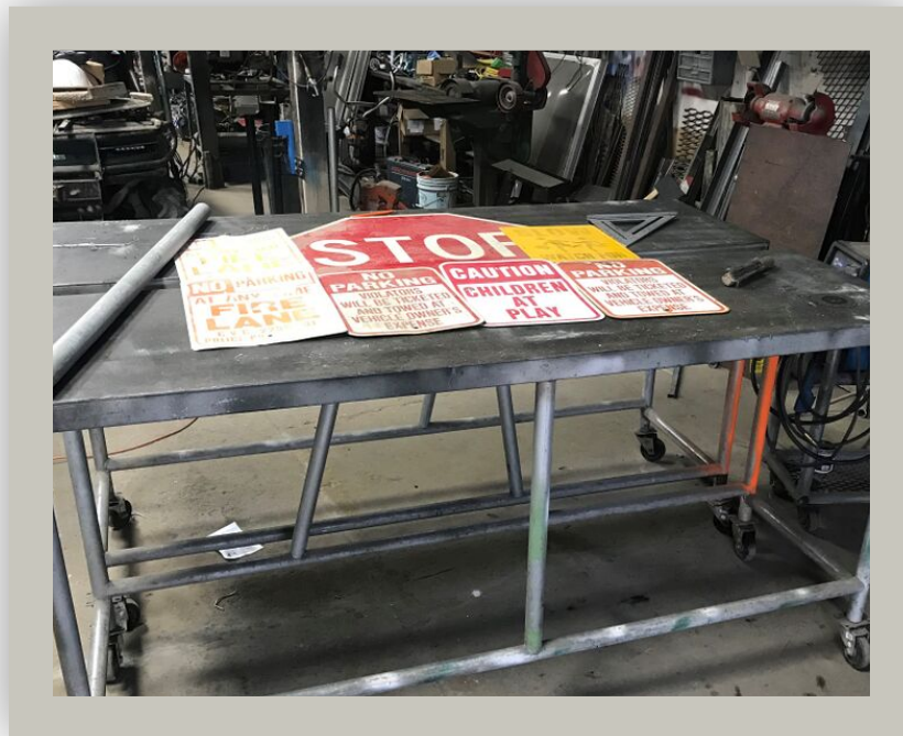
Figure 55 Some materials needed to construct an upcycled street sign bench. By Hayden Miller.
