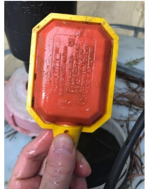
Figure D-1. Sensor Sump Alarm
