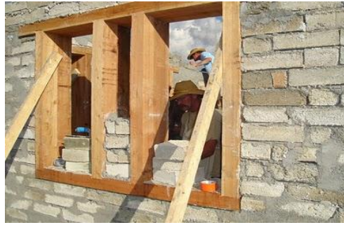
Figure 2.3-2: Papercrete is used to build a structure (Timhp, 2005)
