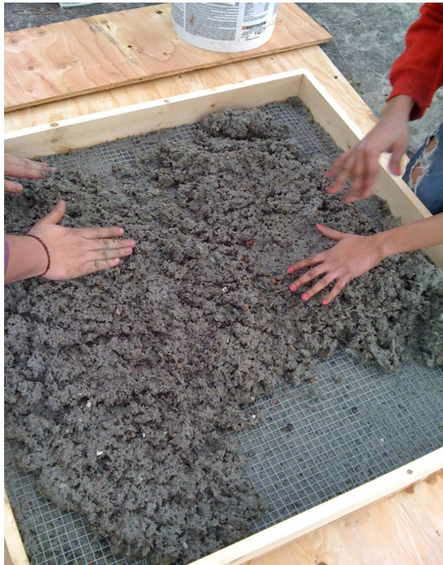
Figure 5 - 3: Here captures the last step of the laying process: setting the second coat of Papercrete (Williams, 2010).
