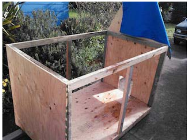
Figure 5.6: Illustrates how the walls are attached to the coop
