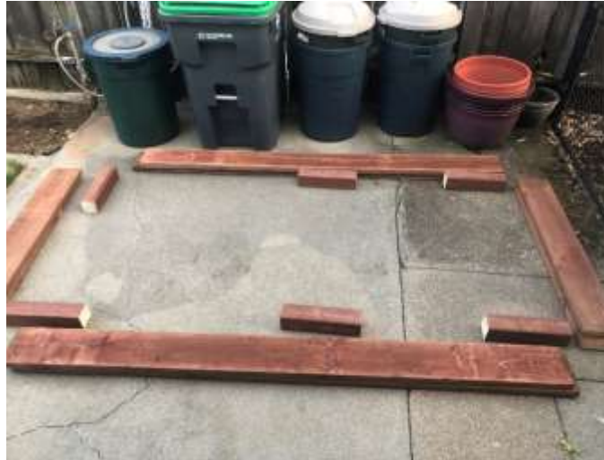
Figure 5-2:Boards Cut to Length
