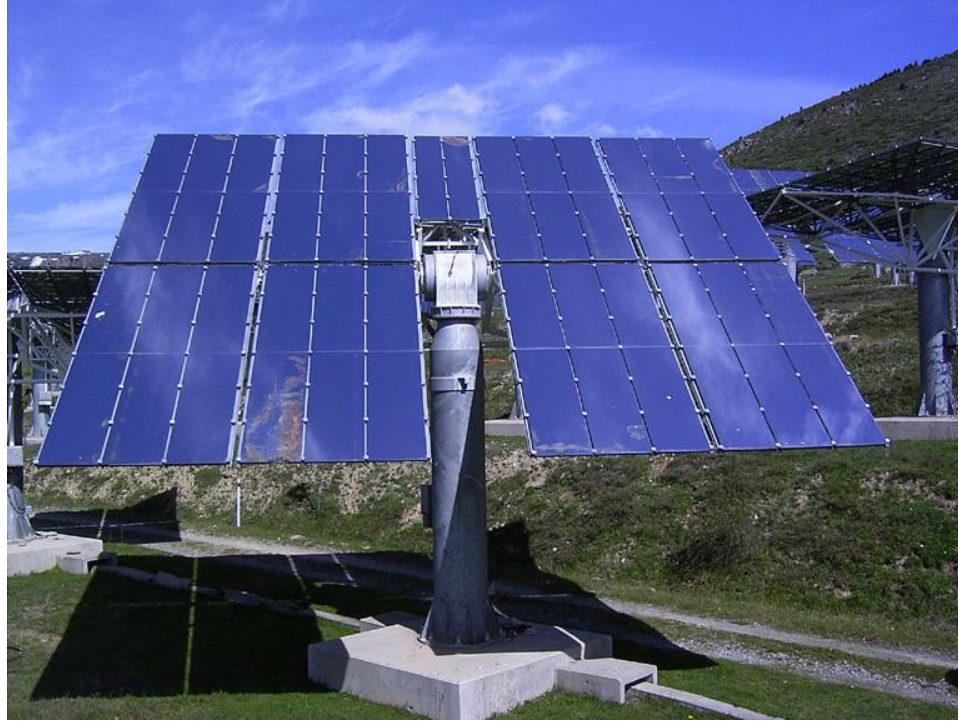
Figure 2-12 Heliostat at Thémis Experimental Station in France
