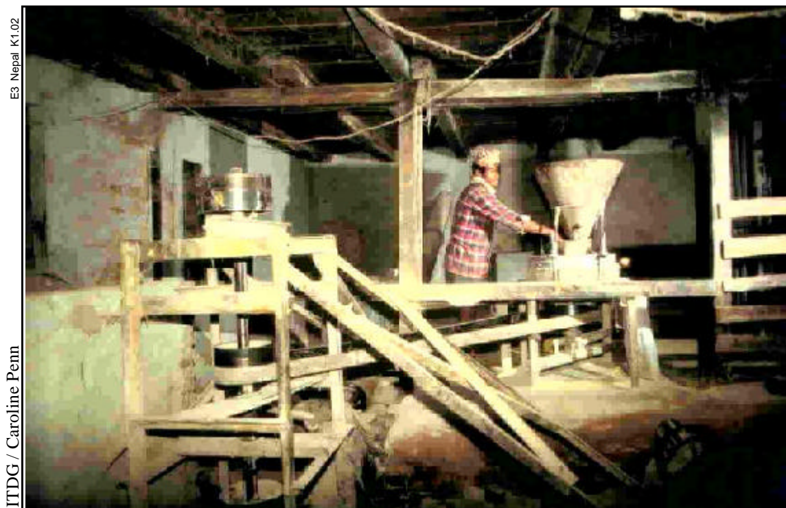
Mechanical energy for grain milling from a micro hydro plant
