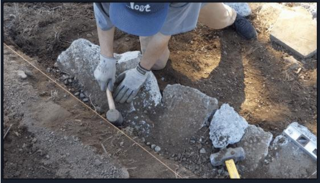
Figure 5-11 Massaging gravel and soil backfill into place
