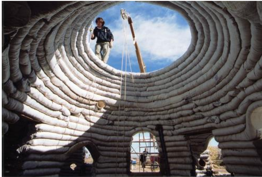
Figure 3-14 SuperAdobe structure in construction (CalEarth n.d.)
