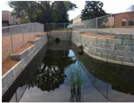
Figure 3-11 Gravity Wall Retention Pond, Plymouth, MN (ReCon Retaining Walls, n.d.)
