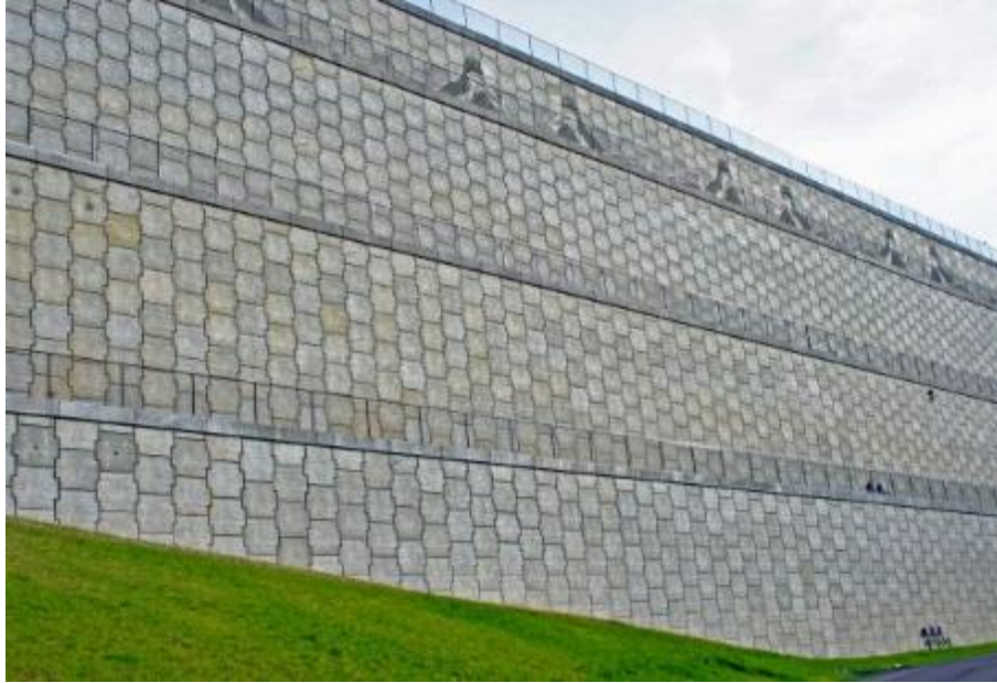
Figure 3-9 Seattle - Tacoma International Airport MSE Wall (Reinforced Earth 2019)
