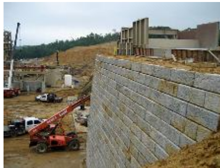
Figure 3-12 Blair Quarry Reinforced Gravity Retaining Wall, Blair, WI (ReCon Retaining Walls 2011)
