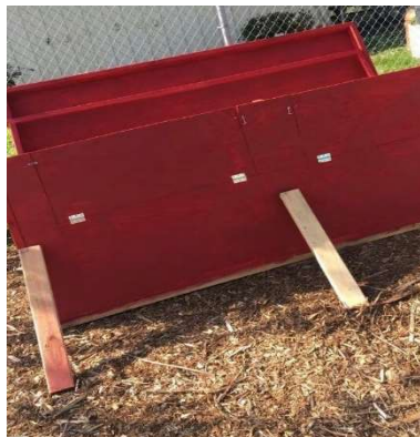
Figure 5-16. Application of weather resistant paint by Ronnel Yabut.
