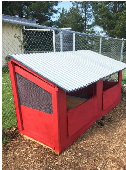
Figure 5-9. The sides of the composter are a combination of wood and hardware cloth. (Ronnell Yabut)
