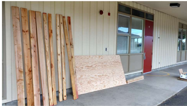
Figure 5-13. Some of the materials bought for the project. By Ronnel Yabut.
