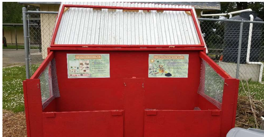
Figure 5-4. The completed composter structure, with doors down and roof up. The educational posters are located on the back wall, as shown. By Kelsey Burrell.
