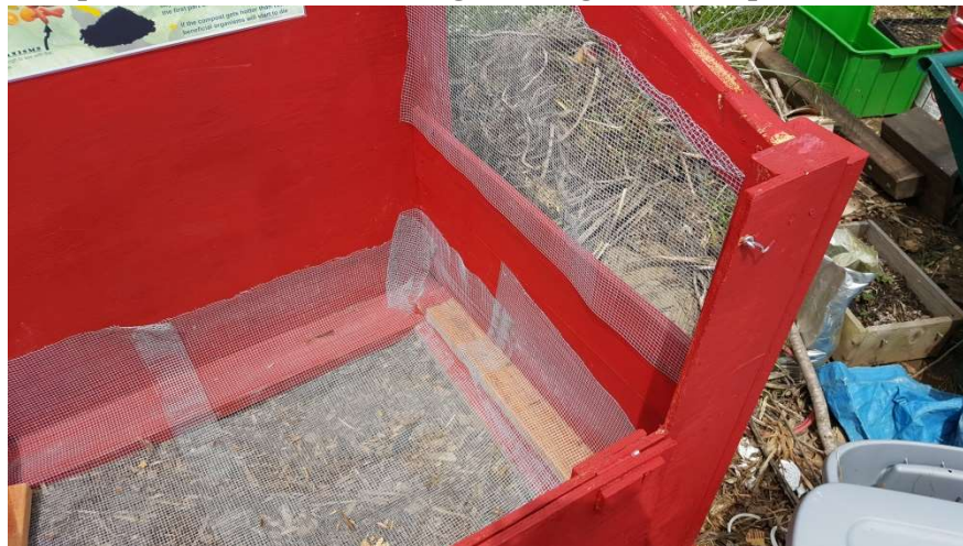
Figure 5-19. Lining the bottom of the compost bins with metal wire. By Ronnel Yabut.
