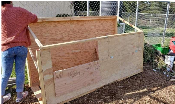
Figure 5-14. Attached doors with hook latches. By Ronnel Yabut.
