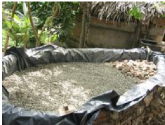
Figure 23: Pond with liner and stone layer: (“Grey water Ecuador La lagrima purificadora” 2012)
