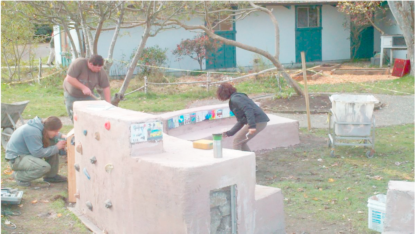
Figure 9 Three Scoops Three Flavors Benches at Laurel Tree Charter School – Earthbag, Urbanite, and Ecoladrillo (“Laurel Tree Charter Schools...”)
