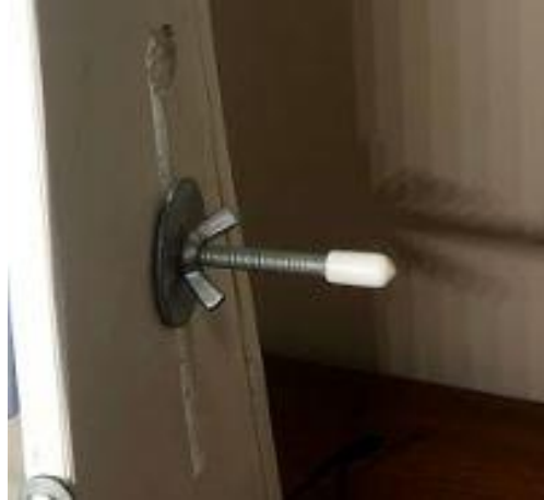
Figure 5.-3 Side of lighthouse. Shows wingnut, washer, and slider handle
