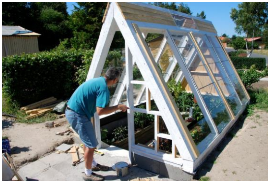
Figure 2.4 A-Frame style greenhouse ( tinyurl.com/p5wjzzh )
