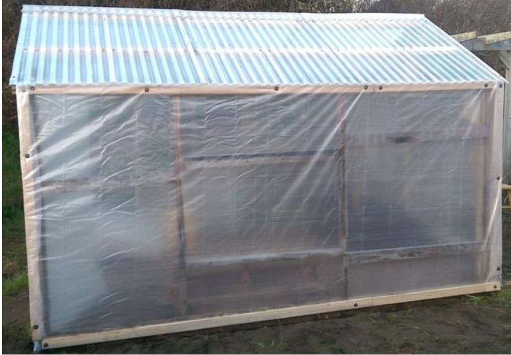
Figure 5.1 South Facing Wall and Roof of Greenhouse. (Photo by: Raymond Rios 11/17/2014)
