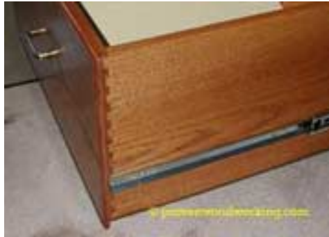
Figure 2-7: Picture of the dovetail. Image from: https://www.wwgoa.com/article/woodworking-joints-which-ones-should-you-use/ .
