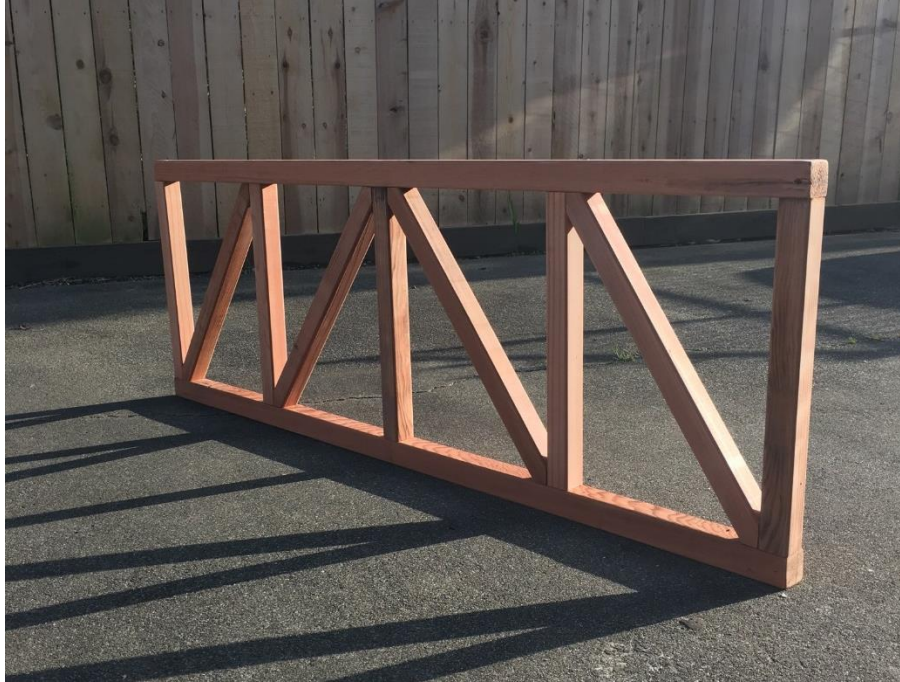
Figure 5.4.3.1: The completed Truss Section.
