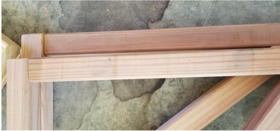
Figure 5.4.4.2: Proper positioning of wing leg on top of the truss section.
