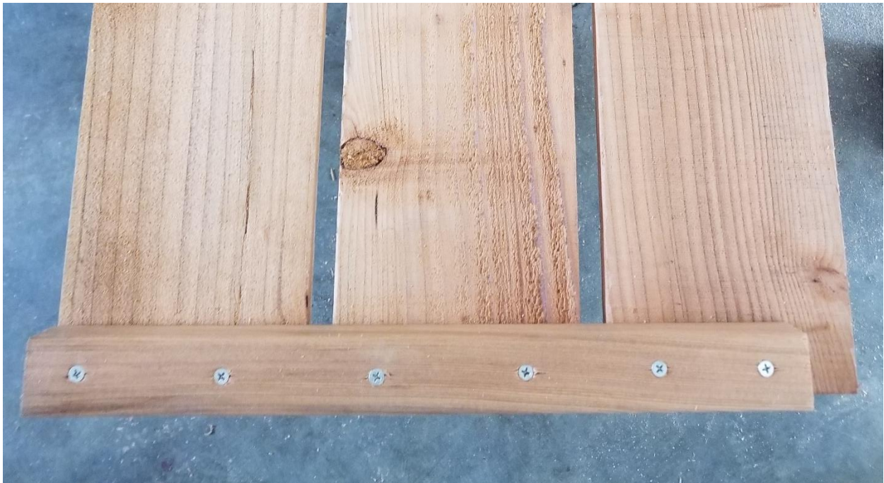
Figure 5.4.1.2: Completion of 2"x2" attachment.
