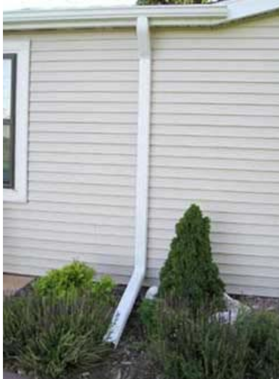
Figure 2-14: Photograph of a typical downspout ( http://www.winnipeg.ca/waterandwaste/drainageflooding/lotGrading/downspouts.stm )
