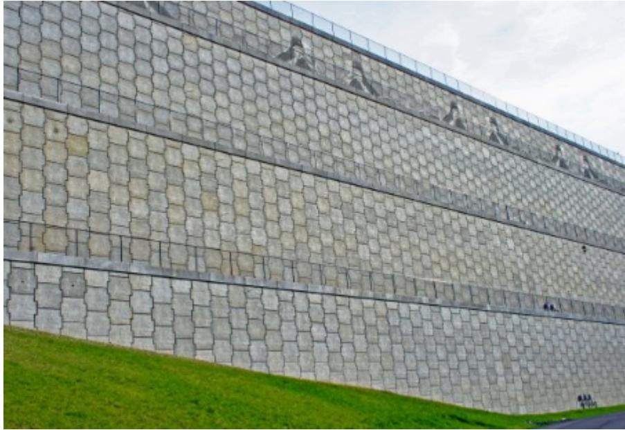
Figure 3-9 Seattle - Tacoma International Airport MSE Wall (Reinforced Earth 2019)
