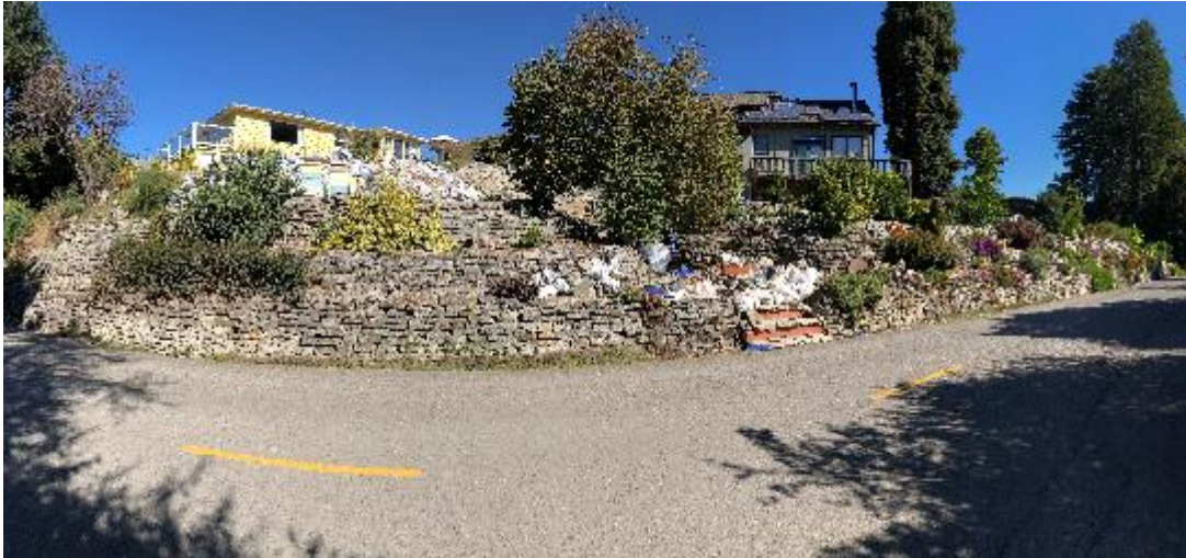
Appendix B 2 Local urbanite construction
