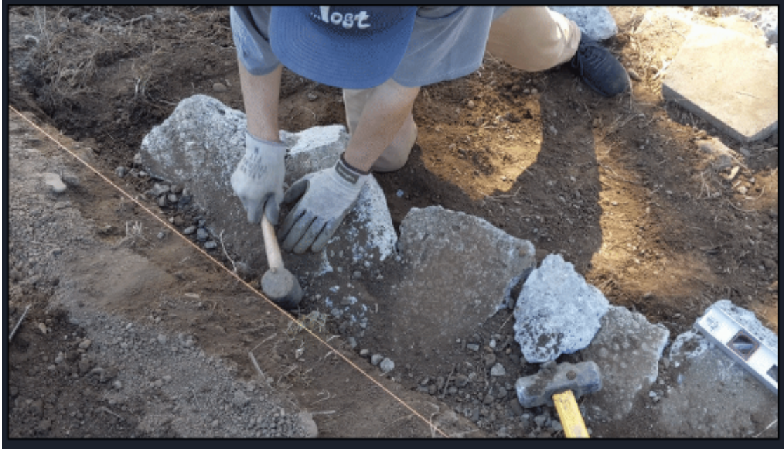
Figure 5-11 Massaging gravel and soil backfill into place
