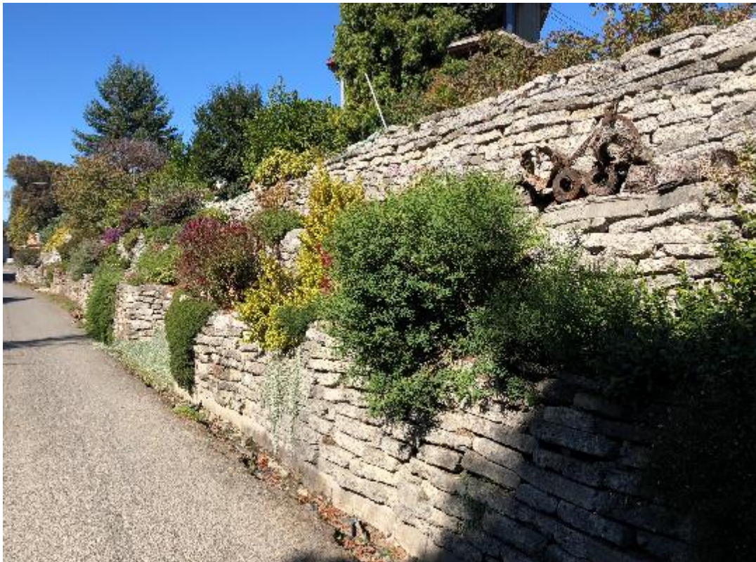
Appendix B 1 Local urbanite construction
