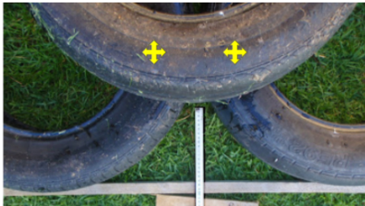
Figure 5-10 Placement of second row of tires.
