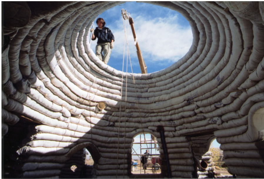
Figure 3-14 SuperAdobe structure in construction (CalEarth n.d.)
