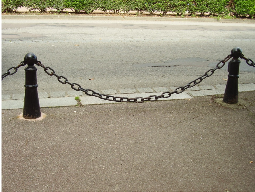
Figure 2.2.4: A catenary curve formed by a hanging chain supported by two posts. ( https://upload.wikimedia.org/wikipedia/commons/0/04/Kette_Kettenkurve_Catenary_2008_PD.JPG )
