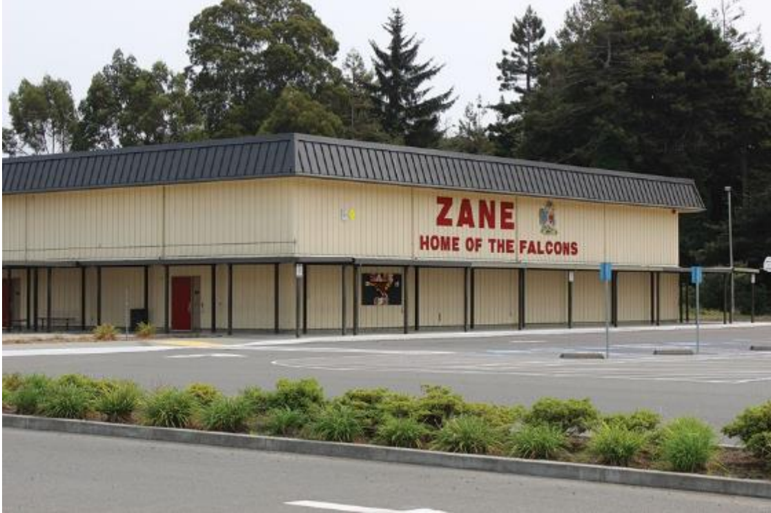
Figure 2-1 Zane Middle School Greenson, T. (2015).
