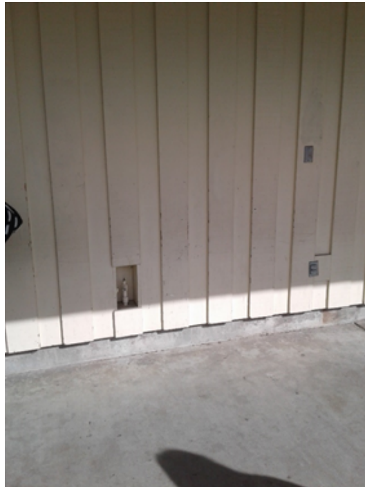
Figure 21: Possible location of small bench outside a classroom at Zane Middle School.
