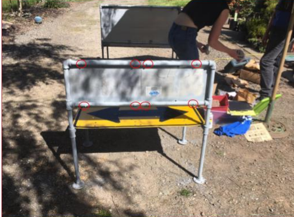
Figure 58: Back of smaller bench with through screws circled in red.
