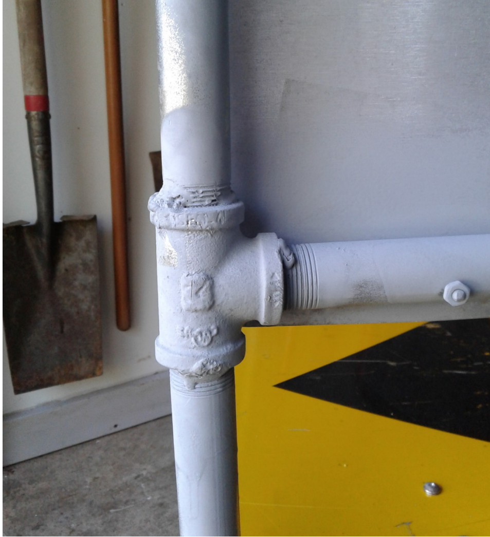
Figure 53: T joint and welds.
