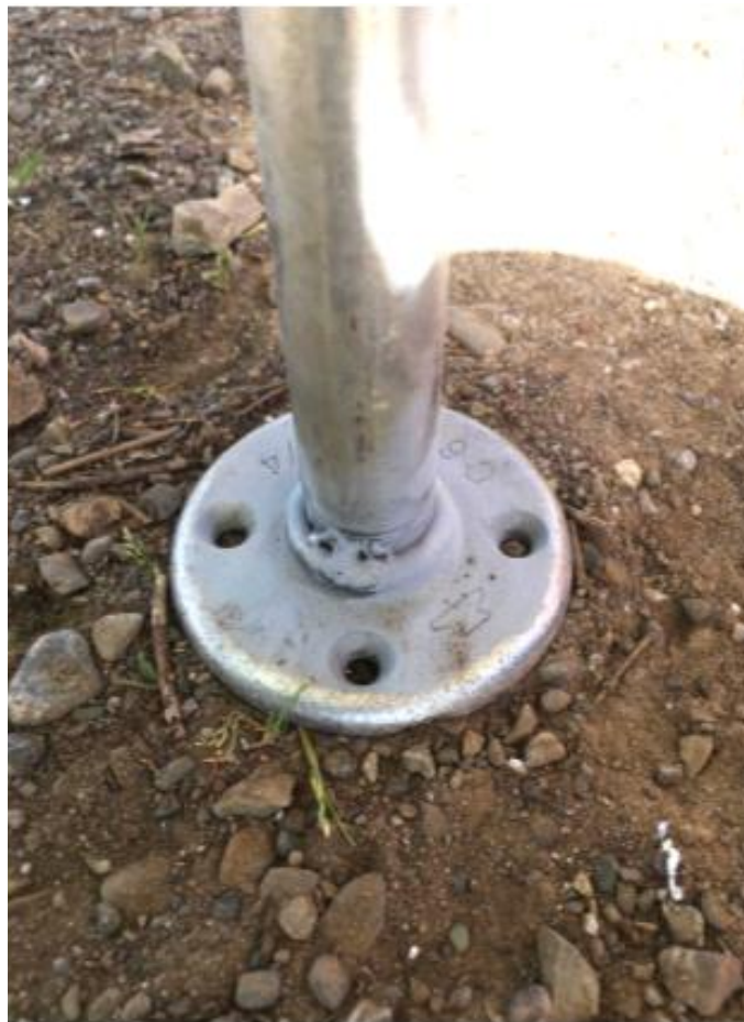
Figure 51: Flange on one of the legs with holes for it to be bolted down.
