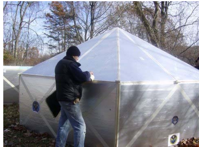
Taping roof section to walls for 12' hexayurt
