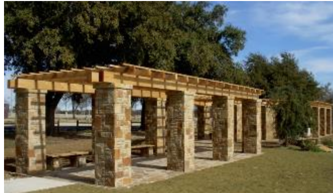
Figure 2.2.10.2: Renovated Pergola at Kiest Park in Dallas, Texas
