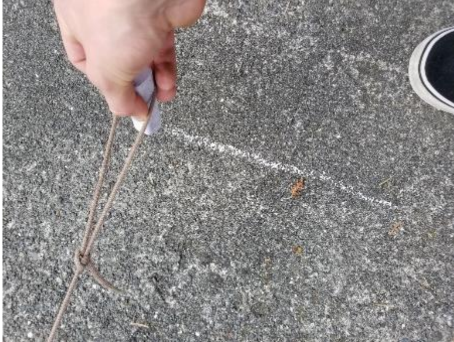
Figure 5.4.5.5: Proper chalk-marking of the circular layout.
