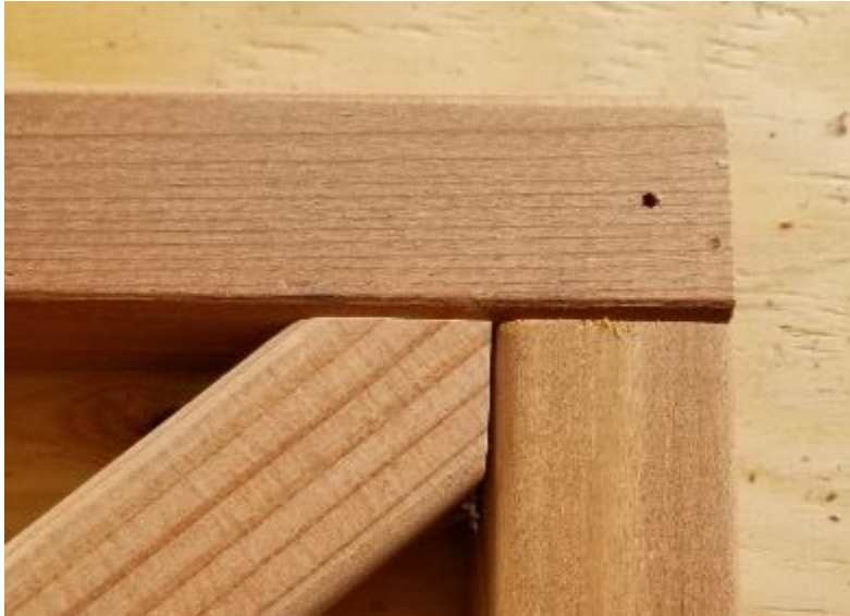
Figure 5.4.2.3: Proper installation of a cross-member joint, and perpendicular angle cut.
