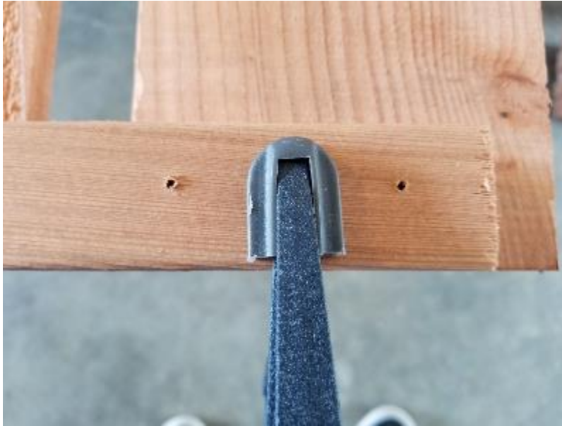
Figure 5.4.1.1: After the first two pilot holes are drilled.
