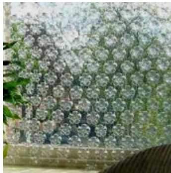
Figure 2.2.11.5: A privacy wall made from interlinking bottoms of plastic bottles (lushome.com).
