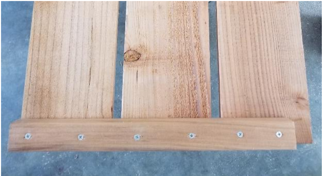
Figure 5.4.1.2: Completion of 2"x2" attachment.
