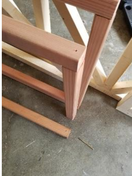
Figure 5.4.2.1: The joint created screwing a 21- \frac{1}{4} " and 15" section together.
