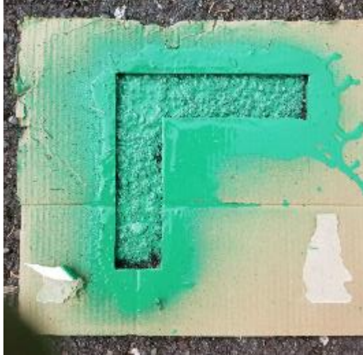
Figure 5.4.5.2: 8"x8"x2" Stencil and painting over the marked chalk.
