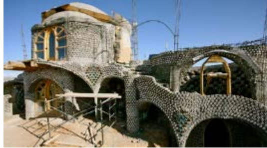
Figure 2.2.11.1: Eve Earthship house construction, made from aluminum cans and adobe.
