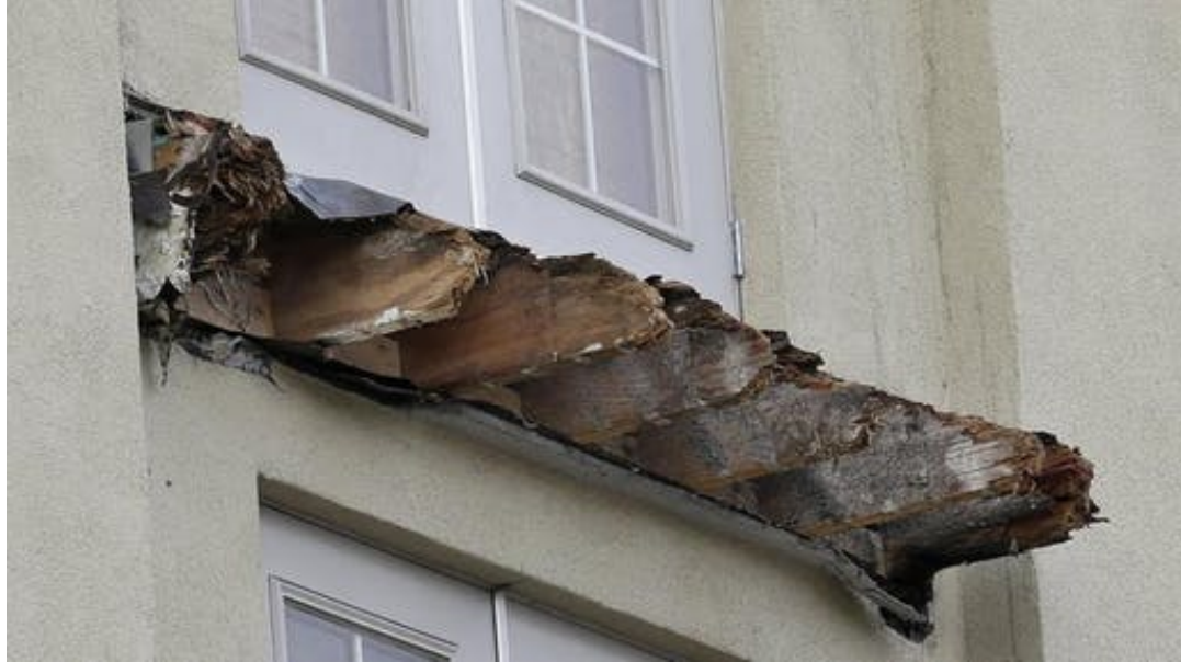
Figure 2.2.8.2: An example of dry rot in wood caused by fungal decay (Archinect.com).
