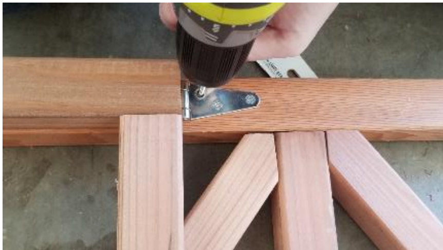
Figure 5.4.4.3: Securing the strap hinge, and wing leg to the truss section.
