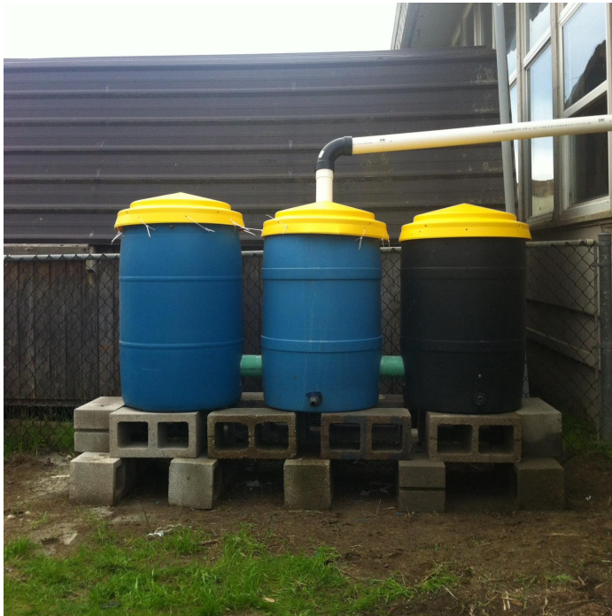
Figure 16: A picture of the completed P.V.C rainwater catchment system taken by the RainBeaus
