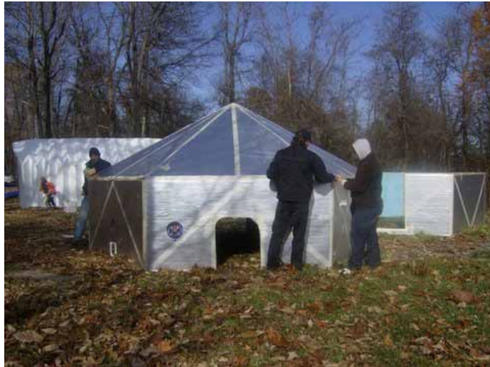
Taping roof section to walls for 12' hexayurt
