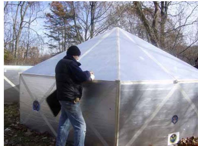
Taping roof section to walls for 12' hexayurt
