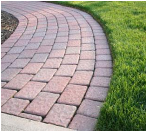
Figure 14: An example of a brick paver walkway (Image Source: http://www.denniscrowley.com/walkways.html )
