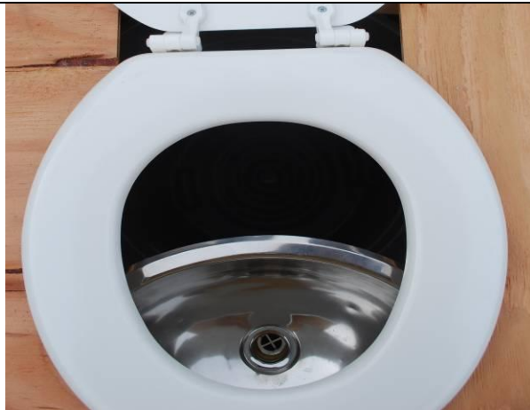
Figure 16 Urine separation view from above. Taken by Ian McBride
