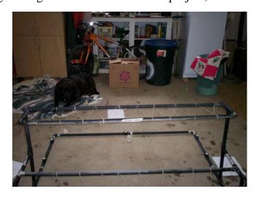
Step 8. Gather pipe sections 12 and 13. Place pipe sections 12 on the backside of the west side of Tier 2. Place pipe section 13 in the same manner, but on the back east side of Tier #2, see Figure 34.
