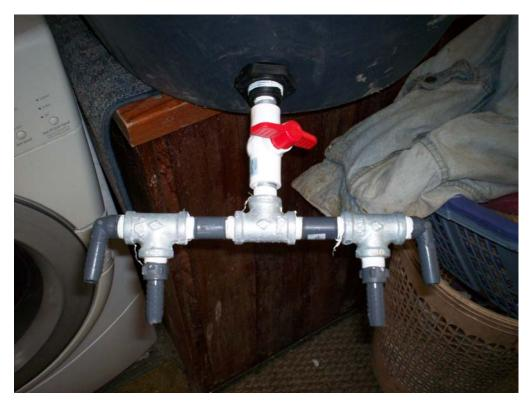
Figure 17: Four-way hose splitter attached to 55-gallon drum.
