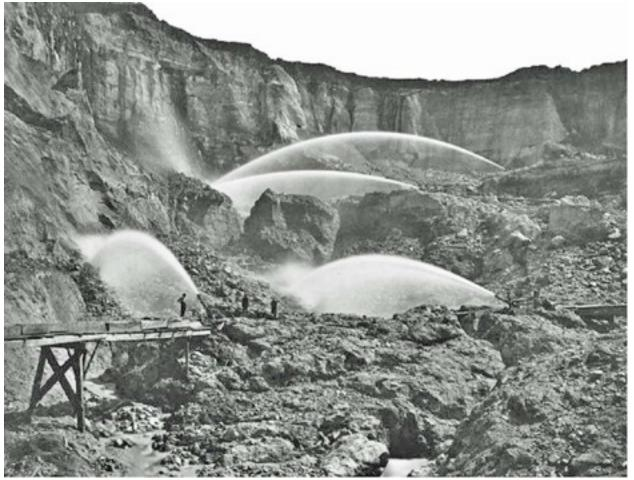
This image shows the use of Hydraulic cannons being used for mining in the 1800's. The same principals that power these cannons can be used to get more force out of a given volume to power a turbine.
