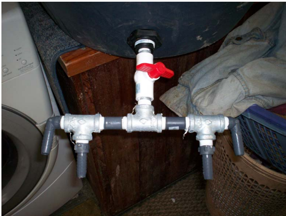
Figure 17: Four-way hose splitter attached to 55-gallon drum.
