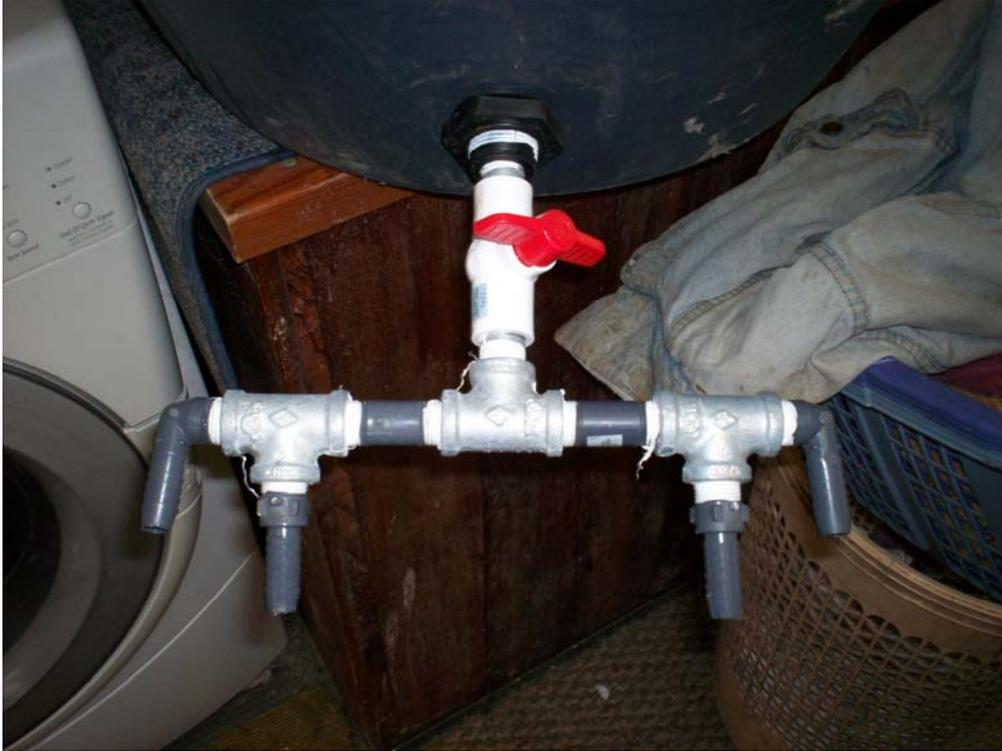
Figure 17: Four-way hose splitter attached to 55-gallon drum.
